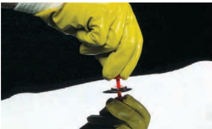
3. Glue the adapter into the dent and align with the cross-mark P.R. = Panel Range
